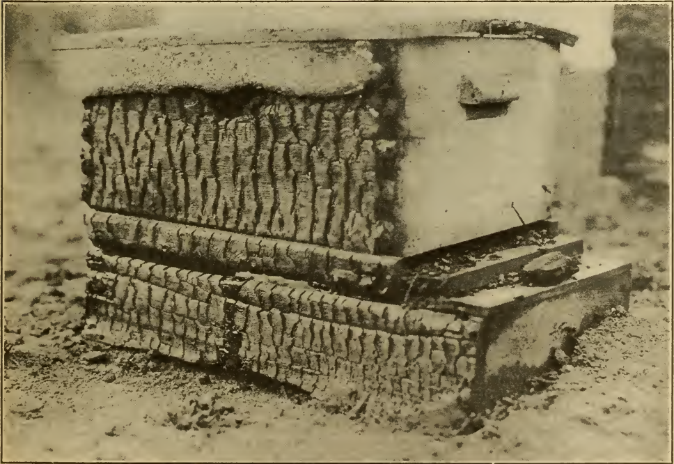
A hive of bees nearly burned up by the heat from an immense lumber yard fire close by. See page 779. Someone threw a pail of water over the hive and put the fire out. During all this heat, the bees, by vigorously fanning with their wings, kept the hive ventilated so that the combs did not melt. Combs made from paraffin or any substitute for beeswax would melt even with the heat of the sun. Beeswax has the highest melting point for its ductility of any wax known.
